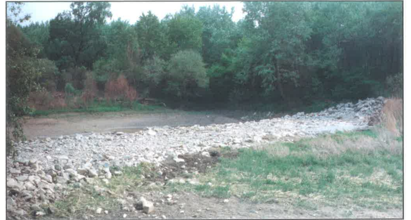
7. A rock-fill transverse structure near the community of Dobrohošť. The bed bottom is covered by old grass suggesting that the branch dried up regularly
