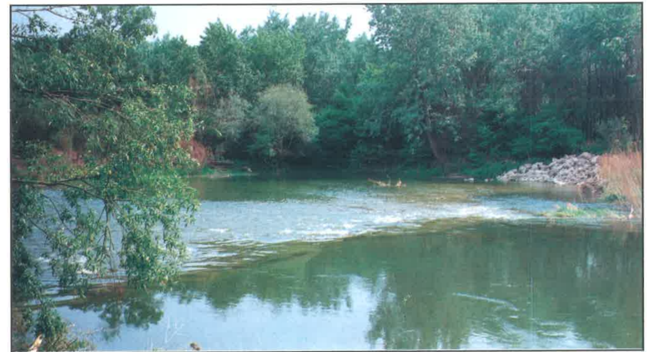
7. A rock-fill transverse structure near the community of Dobrohošť. The bed bottom is covered by old grass suggesting that the branch dried up regularly
