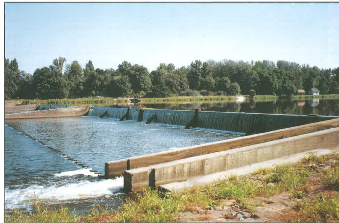
16. A view of the transverse barrage with fish pipeline on the Rhine's old bed at the Rhinau Water Works
