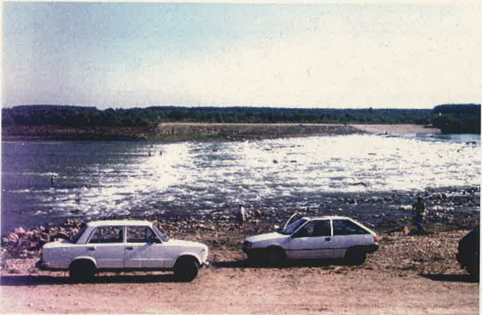
New cross-weir at the Danube near Dunakiliti (rkm 1,842) in July 1995. These rapids are hardly to overcome for most Danube fish.
